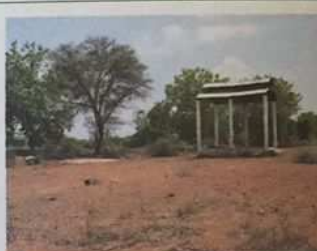
Picture 2: No protection wall at crematorium, Vishnoli (13.06.2017)
